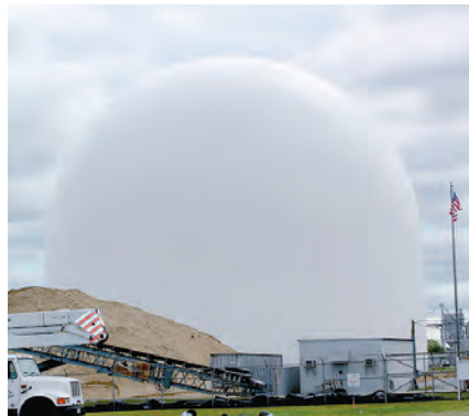
Enviva LP and Dome Technology erected a 157-foot-high storage facility for wood pellets in five hours at the Port of Chesapeake.
