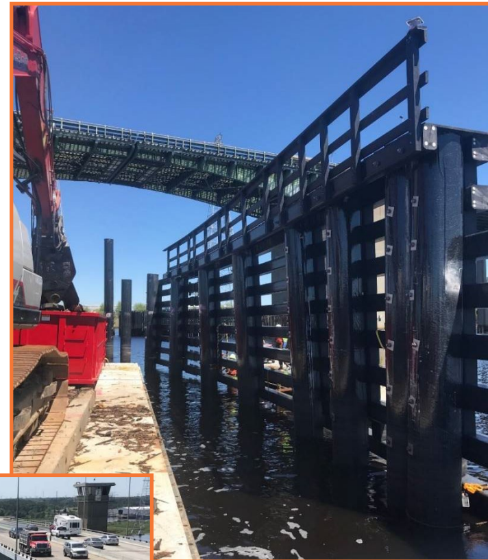
New Fender (Fiber Reinforced Polymer)
