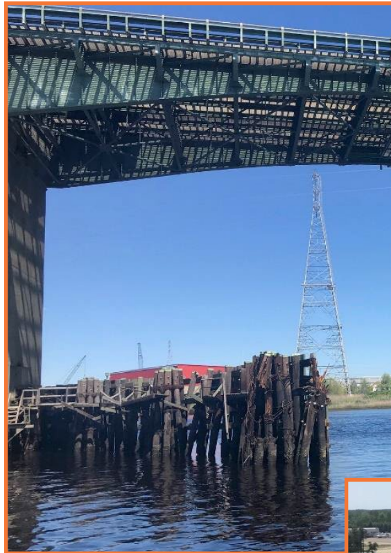
Existing Fender (Timber)
