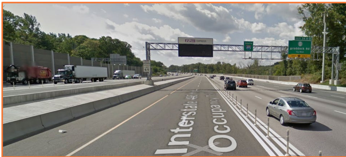
I-495 (Capital Beltway) in Northern Virginia
