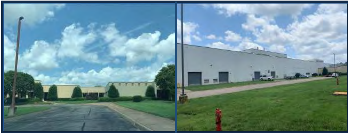
Photograph 1: Views of the front of Building 1.
