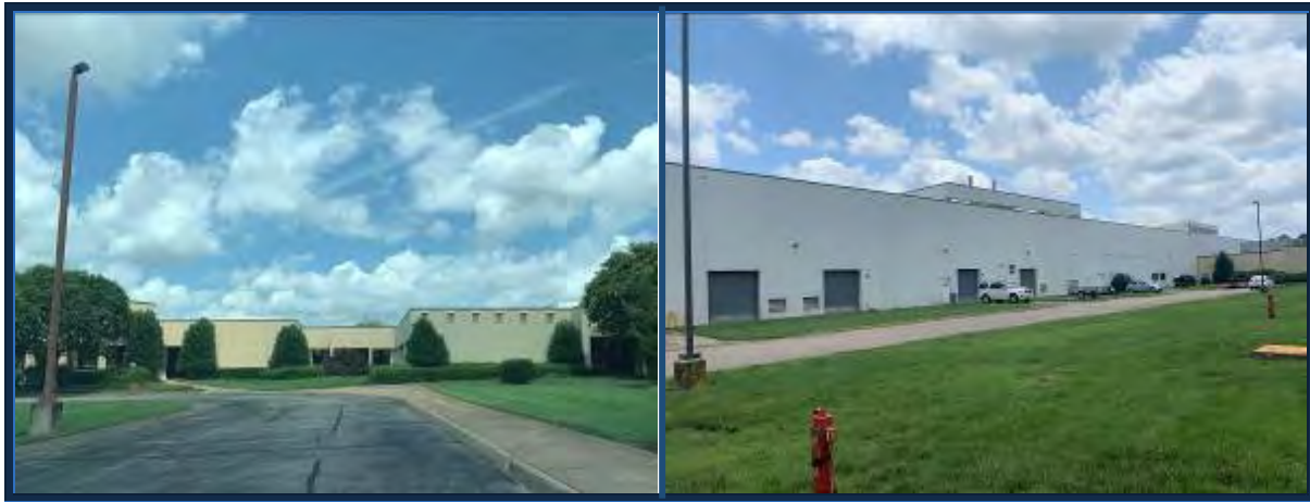
Photograph 1: Views of the front of Building 1.
