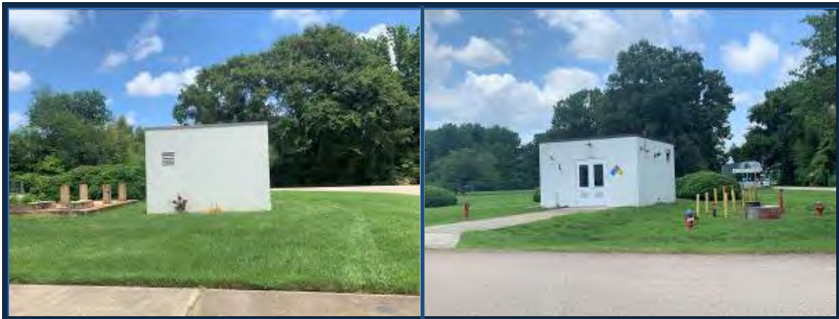
Photograph 5: Views of fire pump houses.
