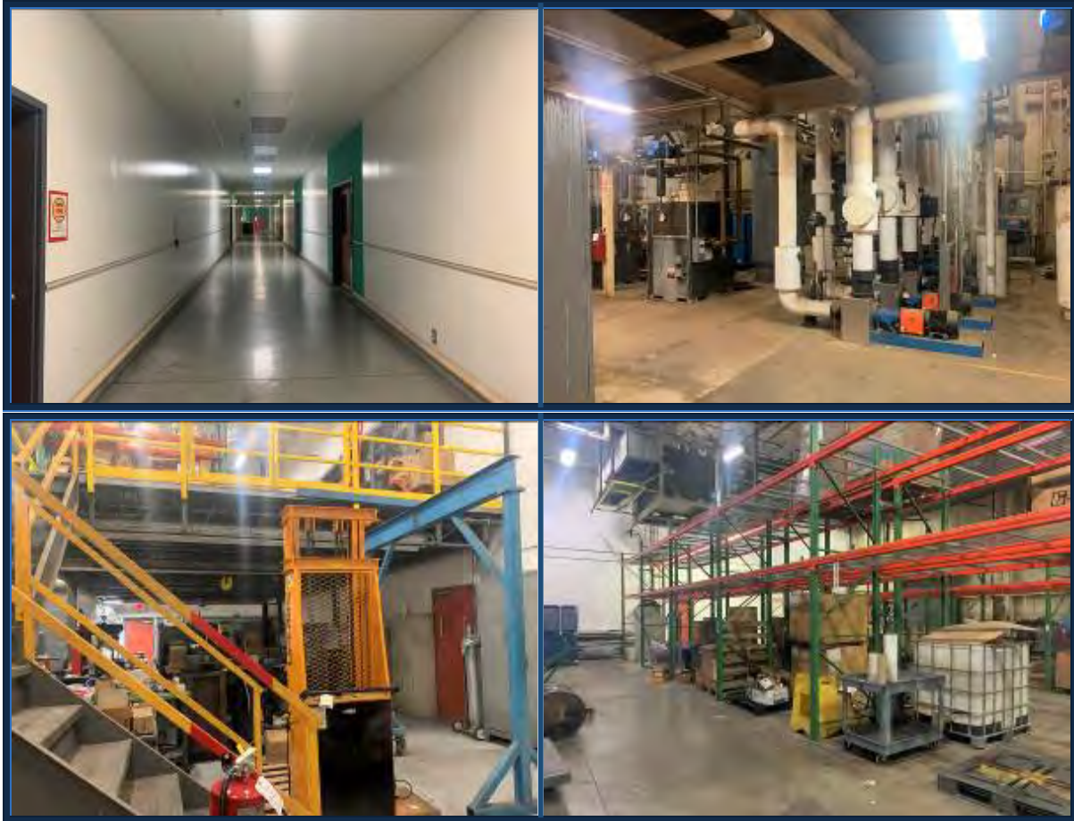
Photograph 4: Representative views of interior industrial spaces (excluding warehouse).
