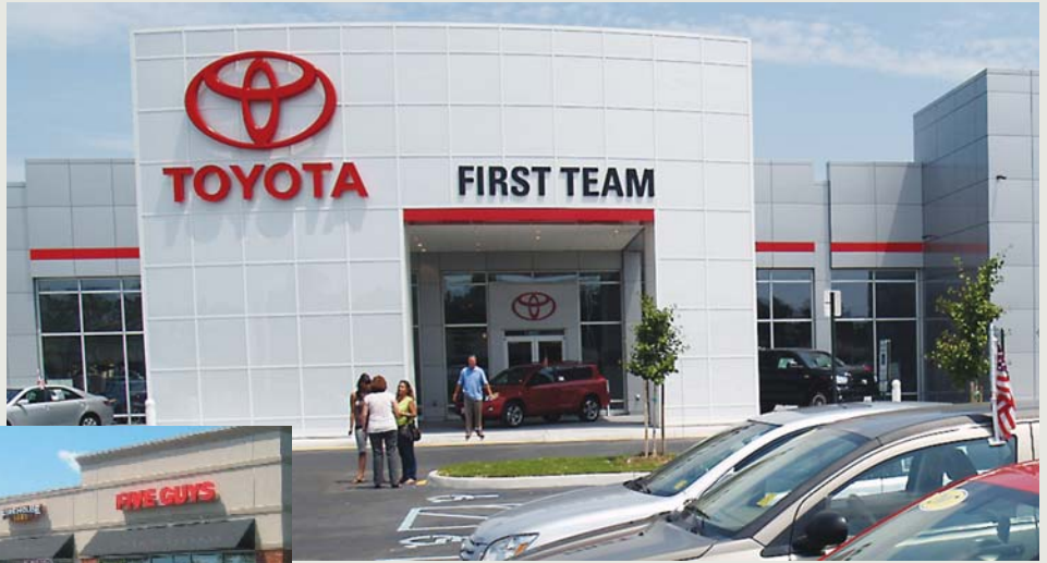
First Automotive Group transformed a former Lowe's on Western Branch Boulevard into one of the largest Toyota showrooms in Virginia and the largest Scion showroom in the U.S. This location serves as First Team's corporate headquarters.
